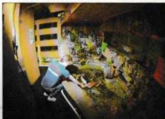
Lynwood Fishhouse - where the Nitra Ghost water treatment system was first imported into Britain.
