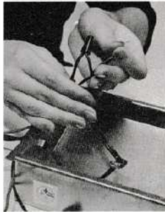
Connect wires with electrical wire nuts included with conversion fixture.
