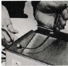
Connect wires with electrical wire nuts included with conversion fixture.
